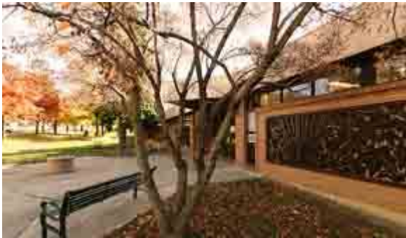
10.2 Toronto Public Library, Amesbury Park Branch. Exterior...
