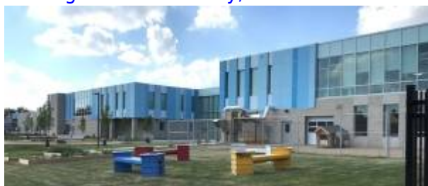
8.2 Regina Public Library, Albert Branch at mâdawêyatitân centre. Exterior...
