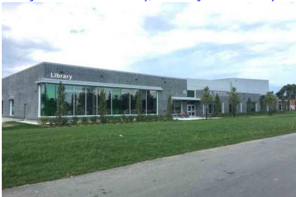
4.2 Kingston-Frontenac Public Library, Rideau Heights Branch. Library Branch and...
