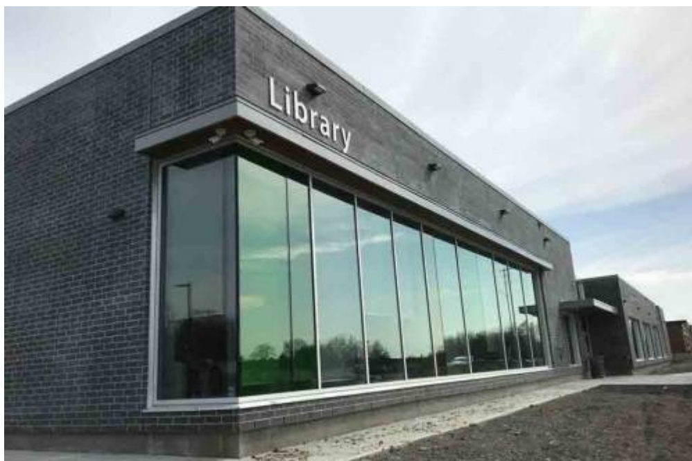
4.1 Kingston-Frontenac Public Library, Rideau Heights Branch. Library Branch and...
