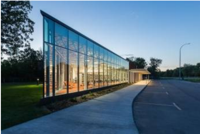
15.4 Winnipeg Public Library, Windsor Park Branch. Exterior at...
