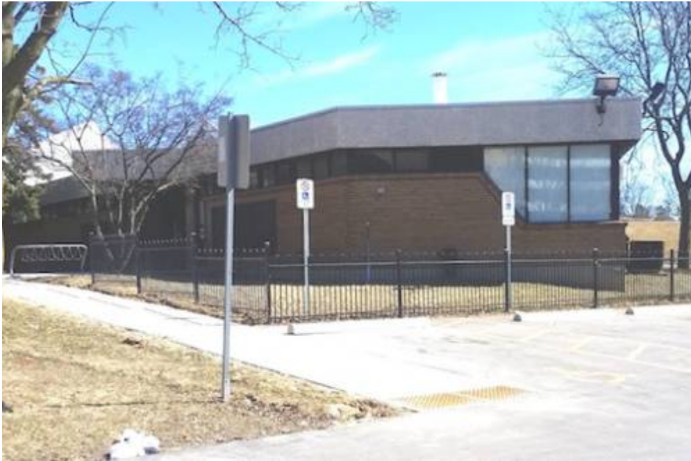
10.1 Toronto Public Library, Amesbury Park Branch. Exterior.Credit.B. Clubb
