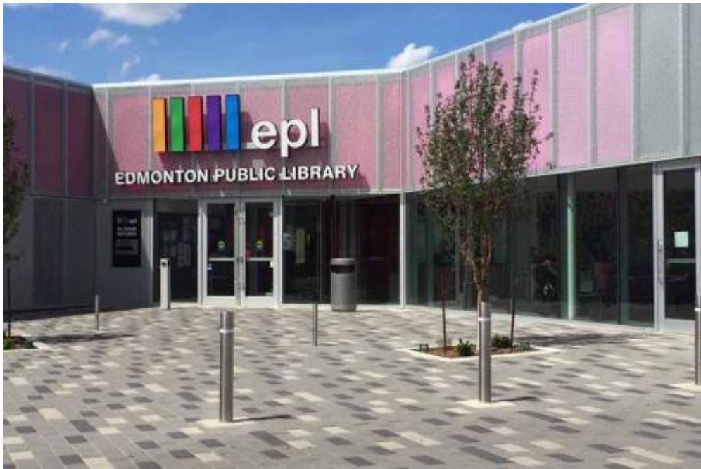
1.1 Edmonton Public Library, Calder Branch. Exterior. Credit Edmonton Public...
