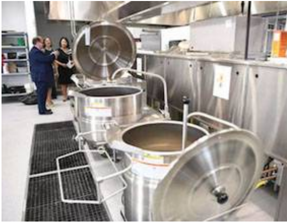
8.13 Regina Public Library, Albert Branch at māmawēyatitān centre.Commercial...
