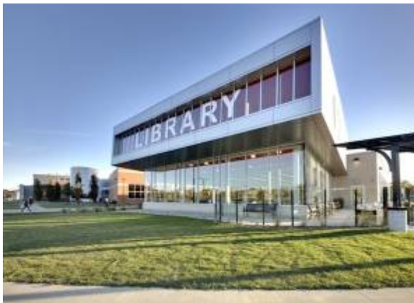
13.1 Vaughan Public Libraries, Pleasant Ridge Branch. Exterior.Credit Peter...
