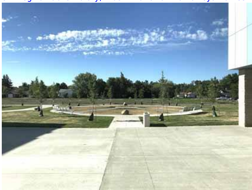
8.3 Regina Public Library, Albert Branch at mâdawêyatitân centre.Exterior....
