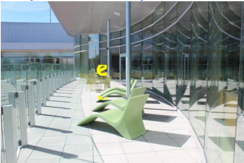
12.6 Vaughan Public Libraries, Vellore Village Branch. Exterior reading...
