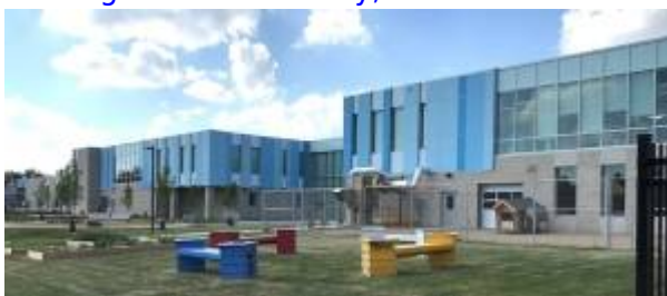
8.2 Regina Public Library, Albert Branch at mâdawêyatitân centre.Exterior...
