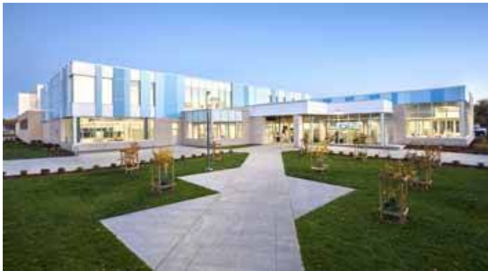
8.1 Regina Public Library, Albert Branch at mâwawêyatitân centre. Exterior....
