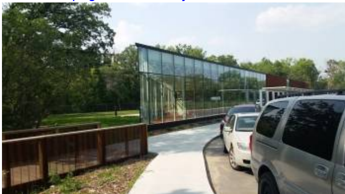
15.2 Winnipeg Public Library, Windsor Park Branch. Exterior, footbridge to...
