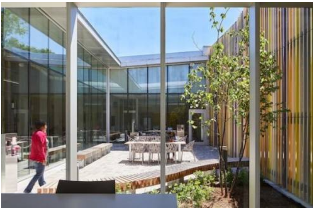
9.6 Toronto Public Library, Albion Branch. External Reading Garden.Credit...
