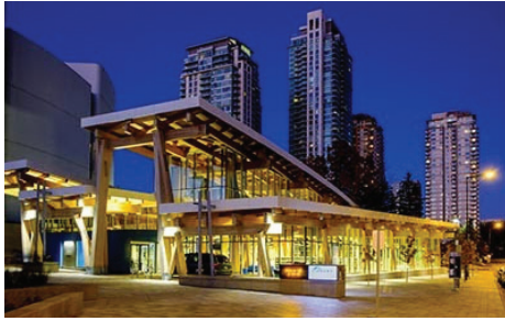
Scarborough Civic Centre Branch, Toronto Public Library
